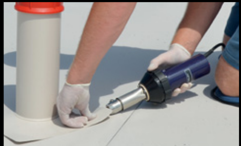
One of various roofing applications.
