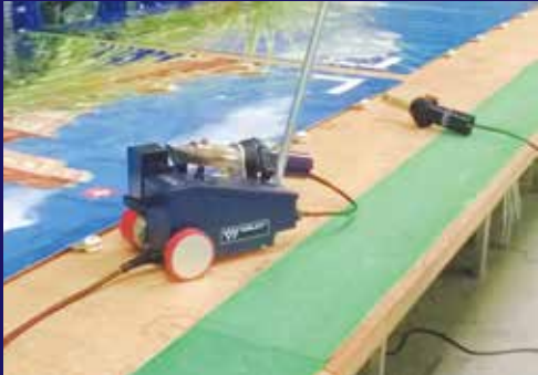
Perfect combination of tarper TW3400 and energy 1600 on site
